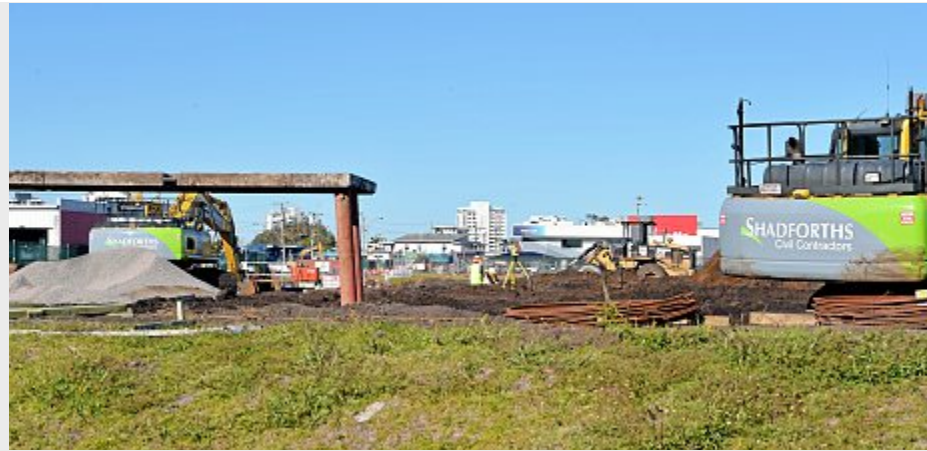
EARTHWORKS: Construction of SunCentral, Maroochydore.
